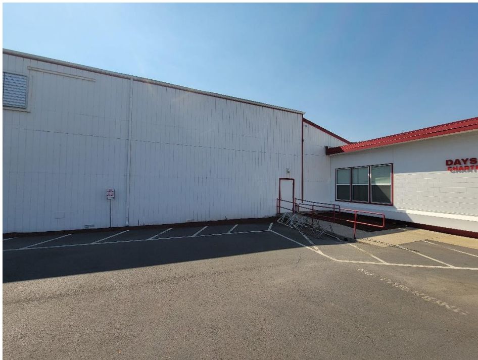
Figure 4: Gymnasium Wall with Connection to Classroom Building
