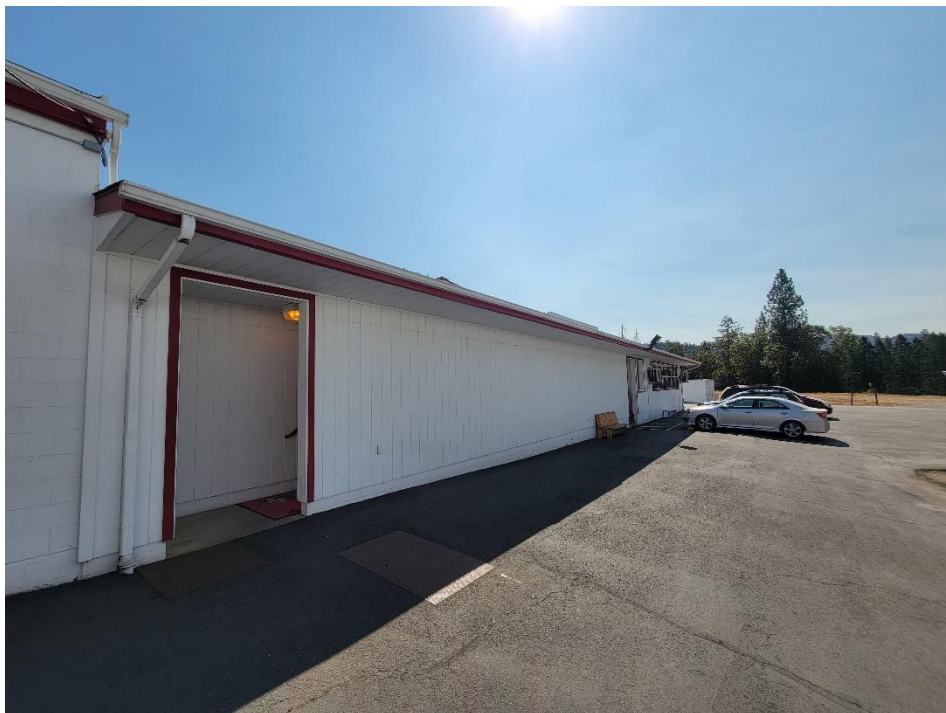
Figure 6: Western Wall of Gymnasium
